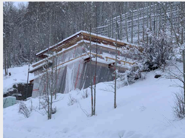
Construction Photo (Winter 2020)
