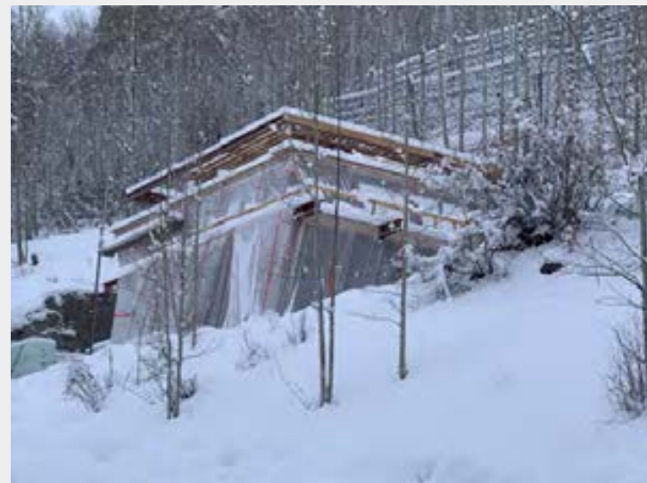
Construction Photo (Winter 2020)
